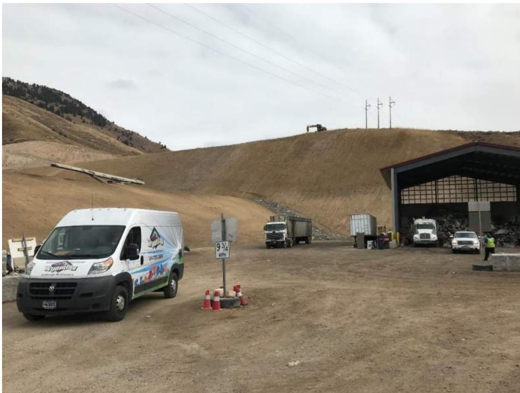
Photo 4. Enhancement areas between Pads 1 and 3 (below power lines) and Pads 1 and 2 (to the left).
