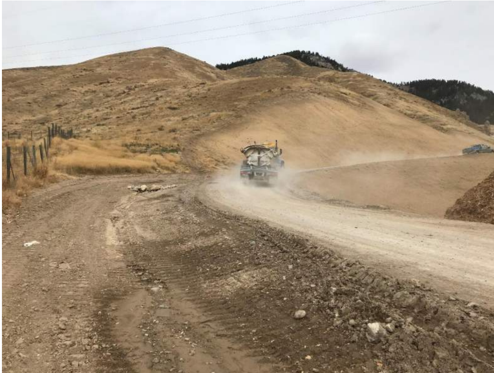
Photo 3. Road to Pad 3, WYDOT property to the west (left).
