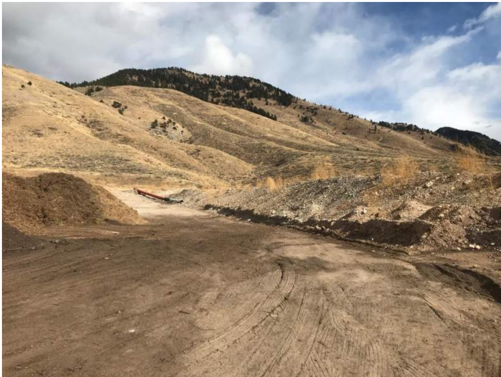
Photo 10. Pad 3 berm stockpiles where it will blend into hillside
