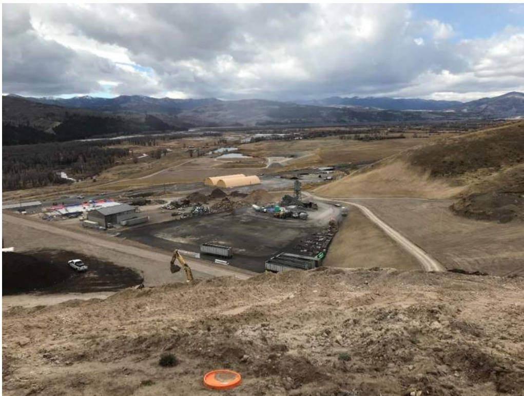
Photo 8. Pad 3, Pad 2 and road between from ridgeline
