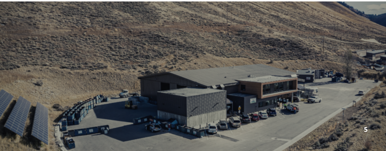
Image 5. Aerial view of the Recycling Center
