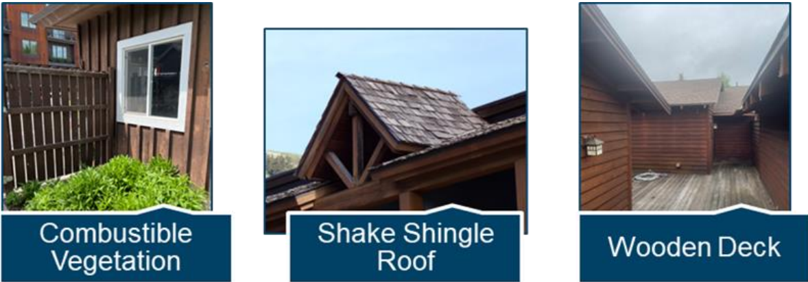
Figure 59: Structure Vulnerability Examples
