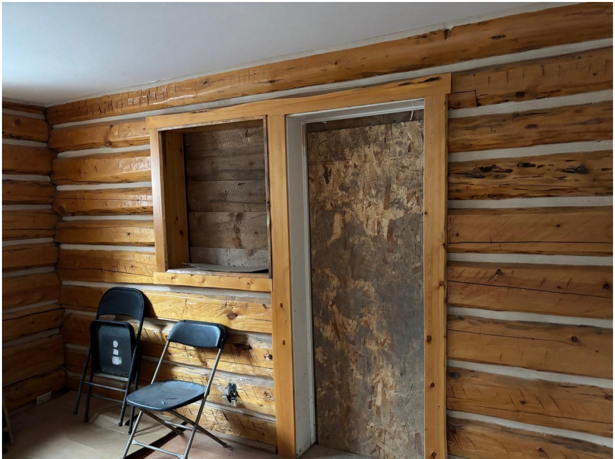
Living Room Back Door Jam with Lead-Based Paint, white
