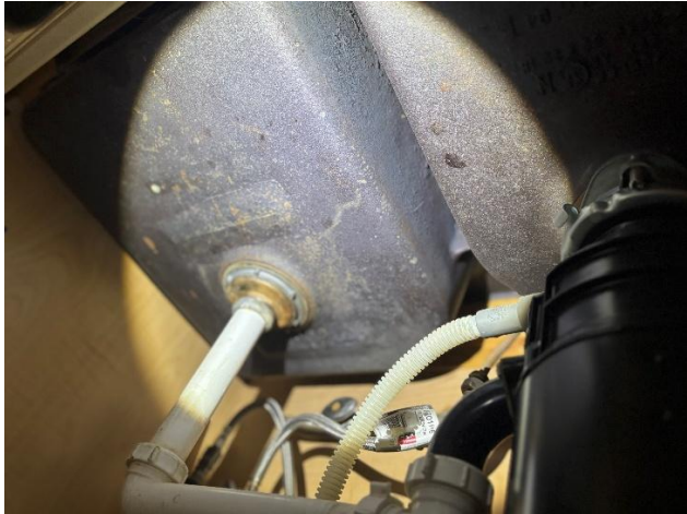
Kitchen Sink Suspected Asbestos Undercoating
