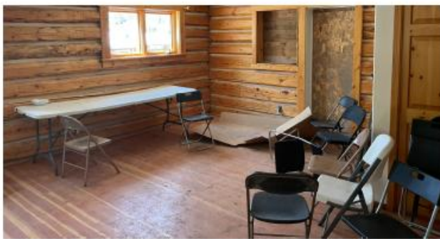
Exposed log walls (with marks) and oak flooring
