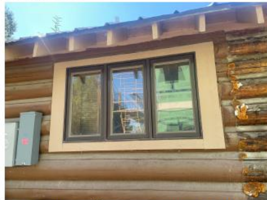
Open eave (N/S eaves), exposed rafter tails, and horizontal fenestration pattern
