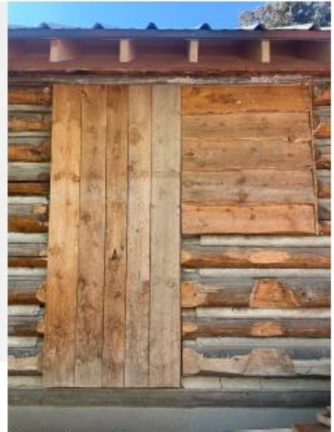
Unfinished logs and unpainted chinking with chinking stops
