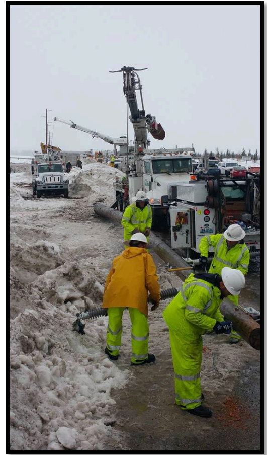
FIGURE 17 - 2017 WINTER STORM; TRANSMISSION POLE BLOW OVER
