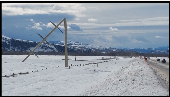
FIGURE 2 – 2017 TETON VILLAGE POWER LINE BLOWDOWN
